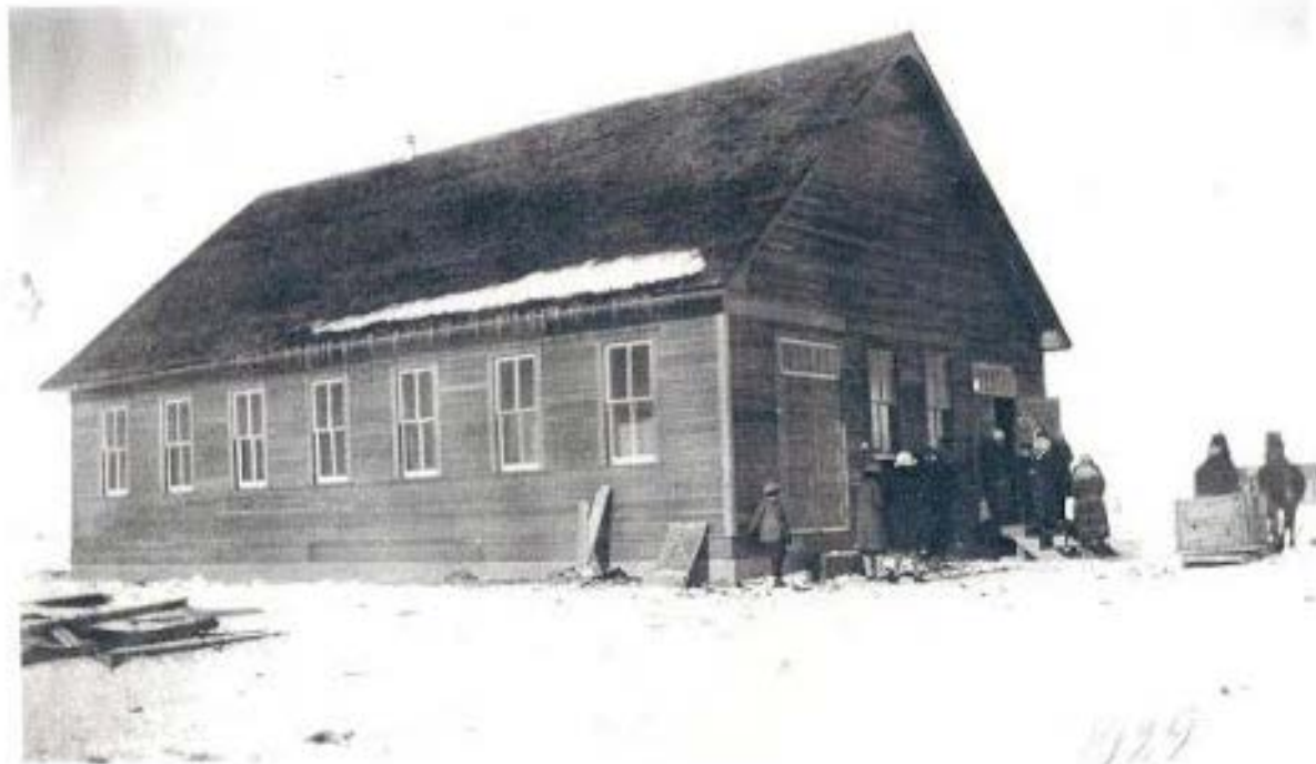
1929 First Coaldale M.B. Church, First Service Jan.25 1929 Construction Start Dec.1928, Thirty-two by Fifty-two Feet
