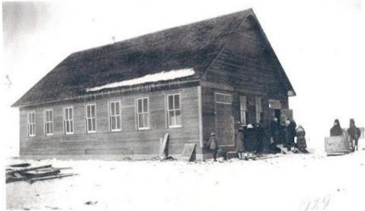
129 First Coaldale M.B. Church, First Service Jan.25 1929 Construction Start Dec.1928, Thirty-two by Fifty-two Feet
